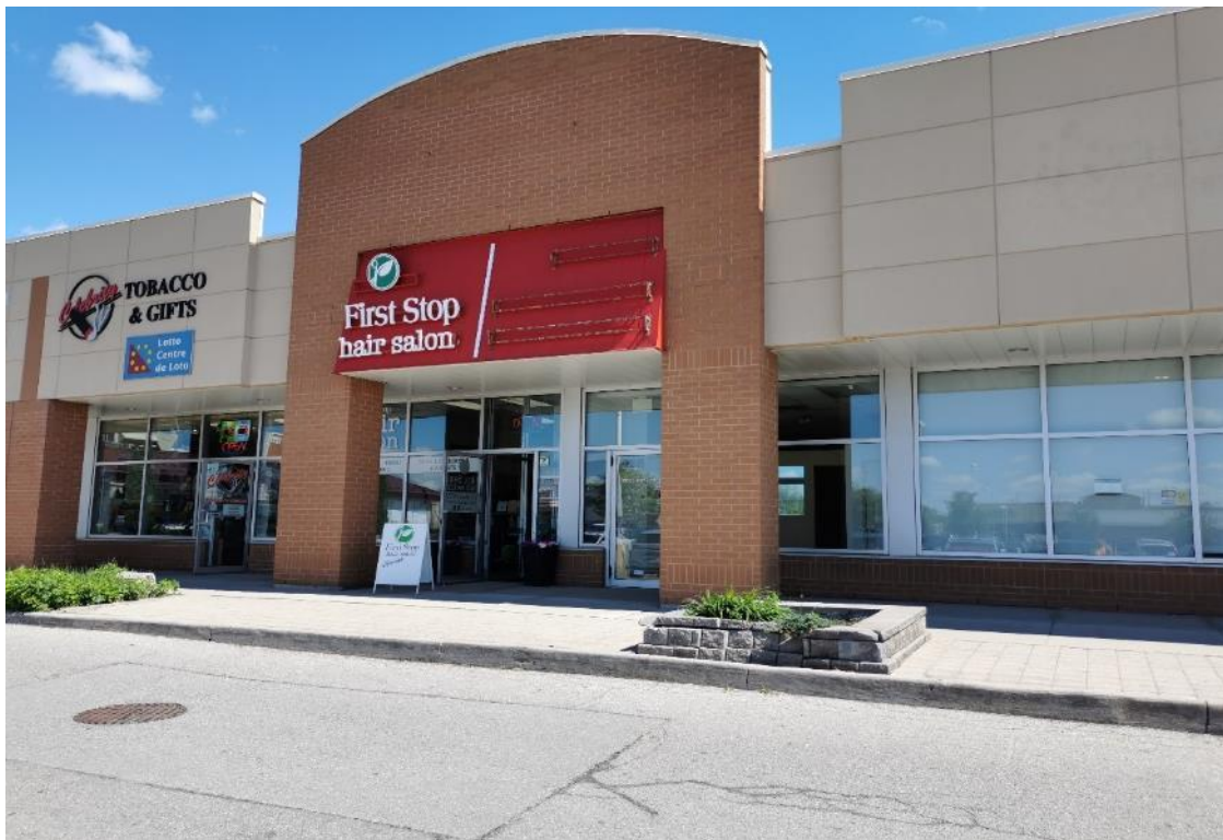
Photo 8: Super Organic Dry Cleaners and Alterations formerly located at 117 Cross Avenue, approximately 60 m southeast, looking northeast.
